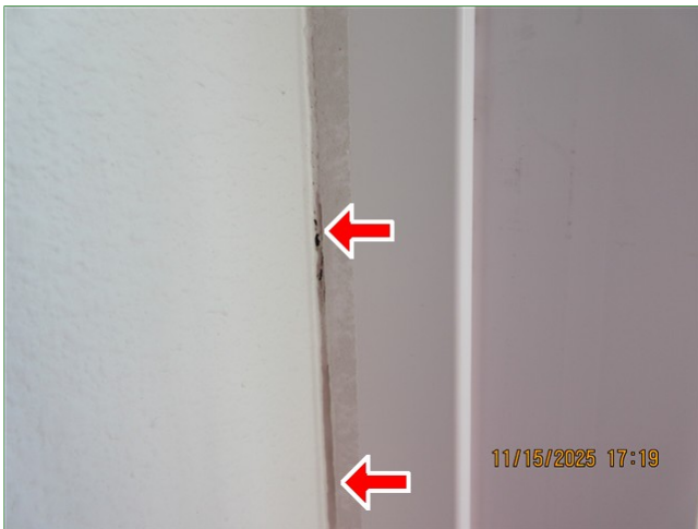
H. Item 3 (Picture) Front of home, window, sealant missing/ separated
