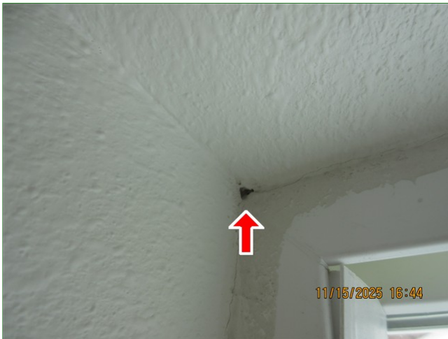
H. Item 2 (Picture) Front of home, window, sealant missing/ separated
