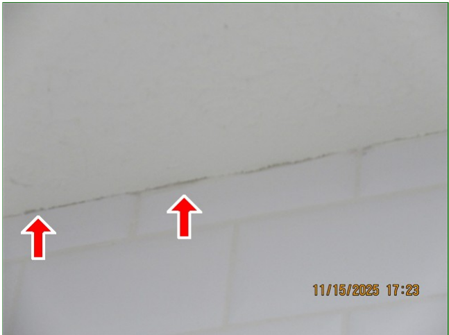
E. Item 9 (Picture) Guest bathroom, tile wall, poor caulk/ sealant work
