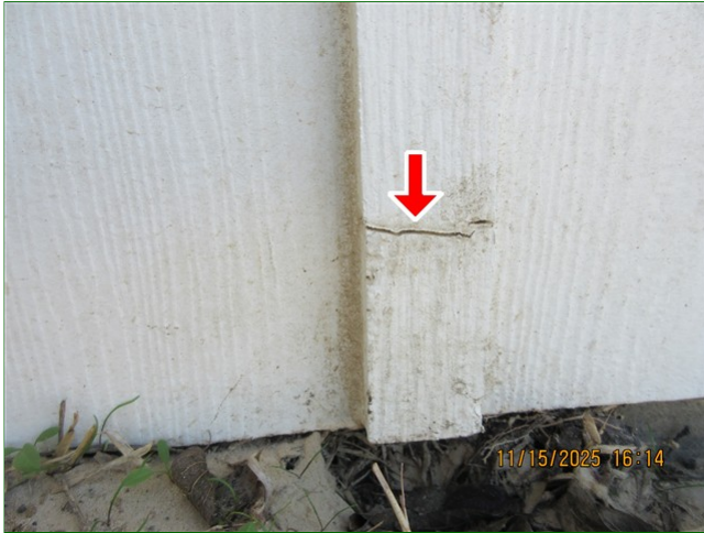
E. Item 22 (Picture) Back of home, siding, damaged
