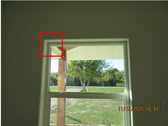
H. Item 1 (Picture) Front of home, window, sealant missing/ separated
