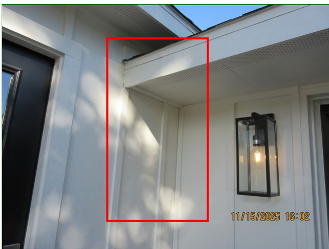
E. Item 2 (Picture) Right of home, roof to wall boards connections, separated caulk/ sealant
