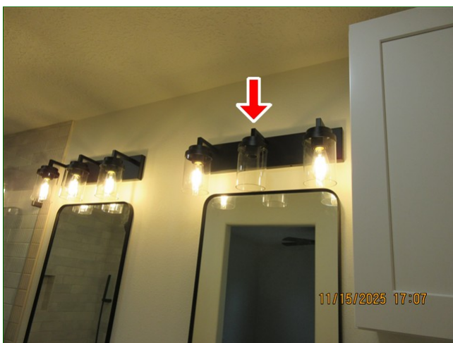
B. Item 3 (Picture) Master bathroom, missing light bulb
