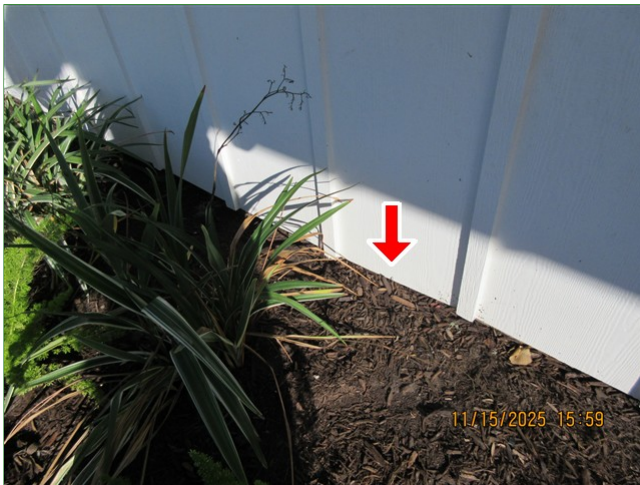
B. Item 4 (Picture) Right of home, high soil/ mulch levels
