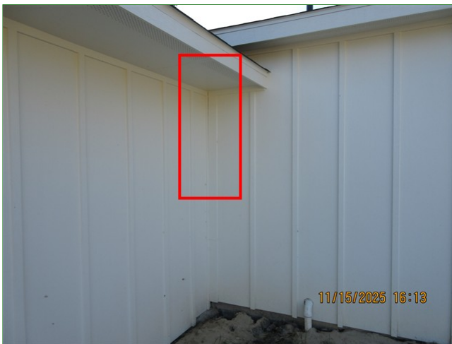
E. Item 17 (Picture) Back of home, siding butt joint, separated
