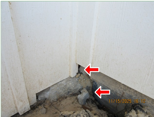
A. Item 2 (Picture) Back of home, foundation, evidence of separate concrete slabs
