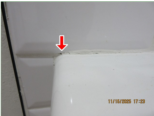
E. Item 32 (Picture) Guest bathroom, tile wall, grout cracked
