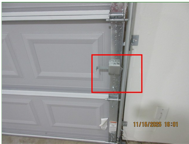
G. Item 1 (Picture) Garage door, manual lock, not disengaged
