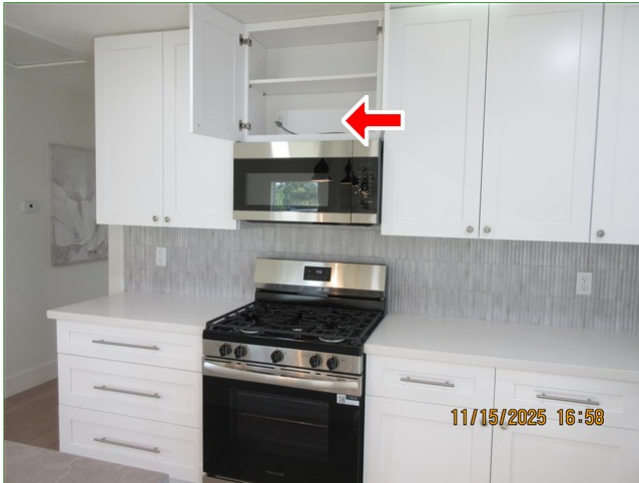
C. Item 1 (Picture) Kitchen, gas fueled oven/ stove, no exhaust vent to outdoors
