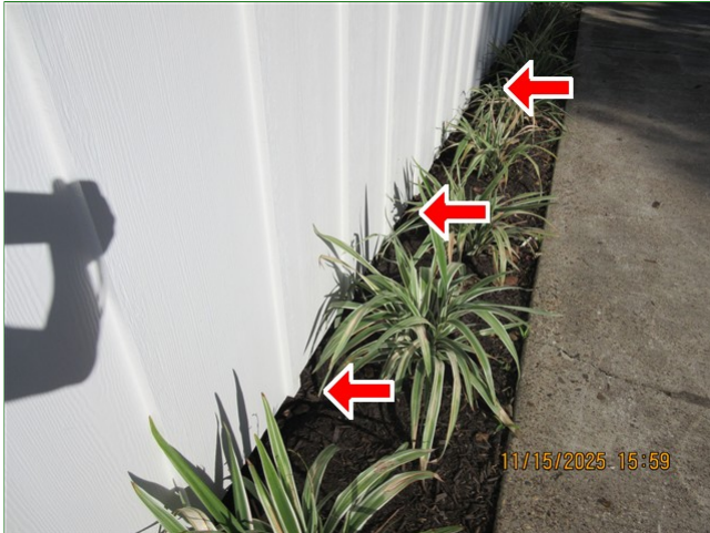
B. Item 3 (Picture) Right of home, high soil/ mulch levels
