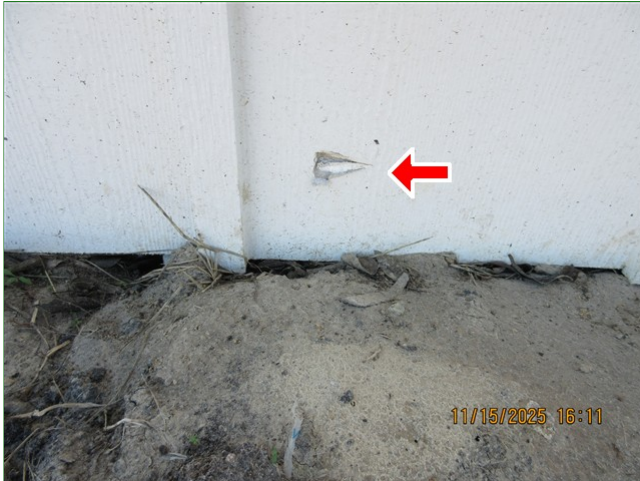
E. Item 16 (Picture) Back of home, siding, damaged
