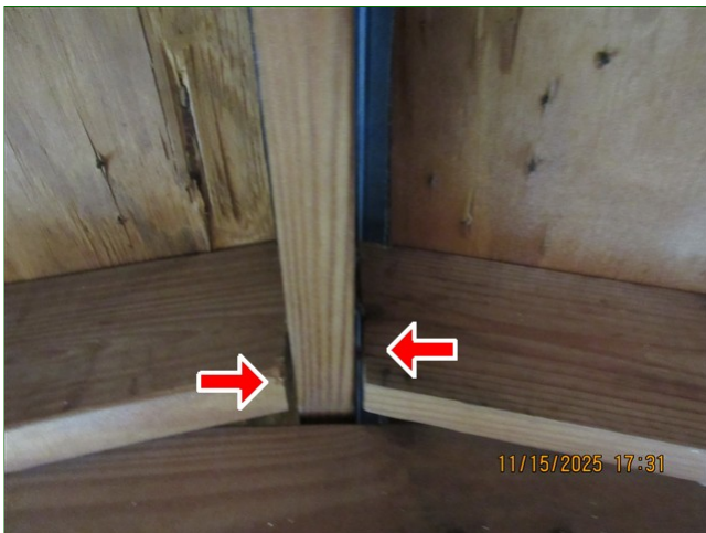
D. Item 2 (Picture) Attic, rafters connection to ridge board, separated
