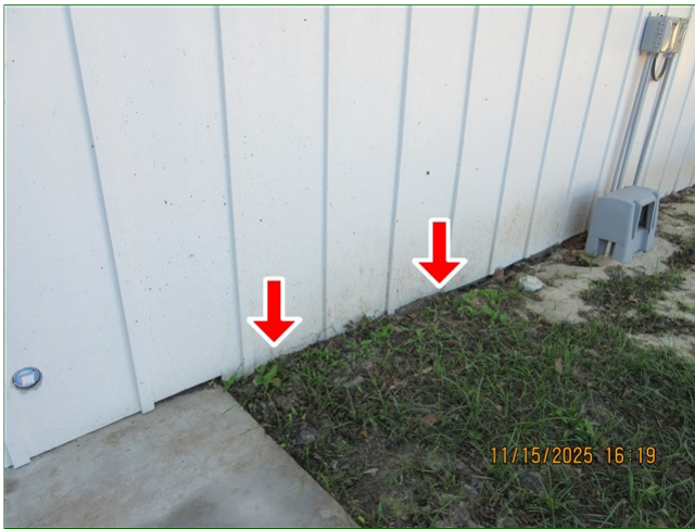
E. Item 23 (Picture) Front of home, cement fiber siding, in direct contact with ground
