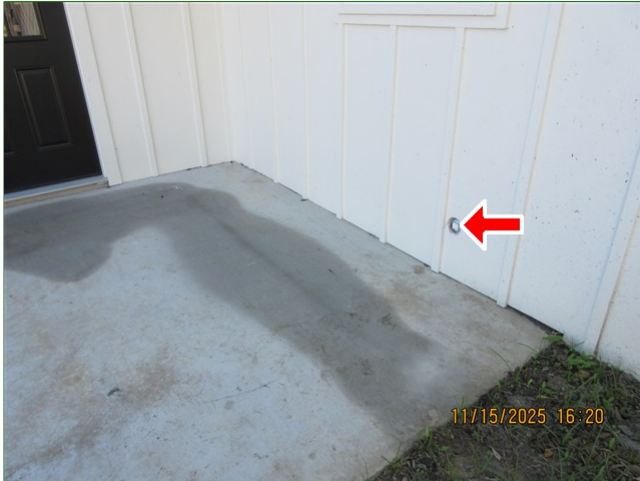
E. Item 24 (Picture) Back of home, through wall termination, no flashing, possible 2 layers of exterior siding
