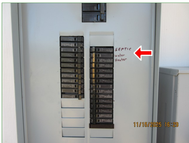
A. Item 1 (Picture) Left of home, panel board, not labeled
