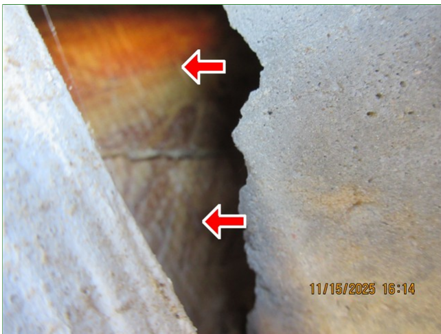
A. Item 4 (Picture) Back of home, foundation, evidence of separate concrete slabs
