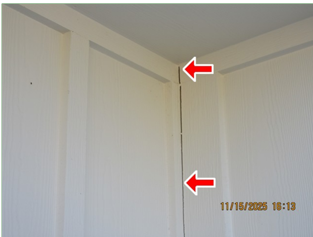
E. Item 18 (Picture) Back of home, siding butt joint, separated
