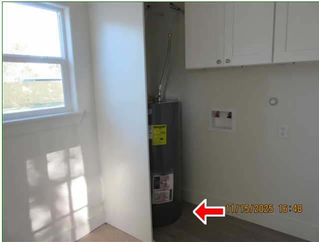
C. Item 1 (Picture) Utility/ laundry room, water heater tank, no auxiliary drain pan or pipe terminating to outdoors
