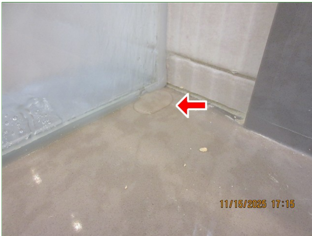
E. Item 30 (Picture) Master bathroom, glass shower wall, missing sealant
