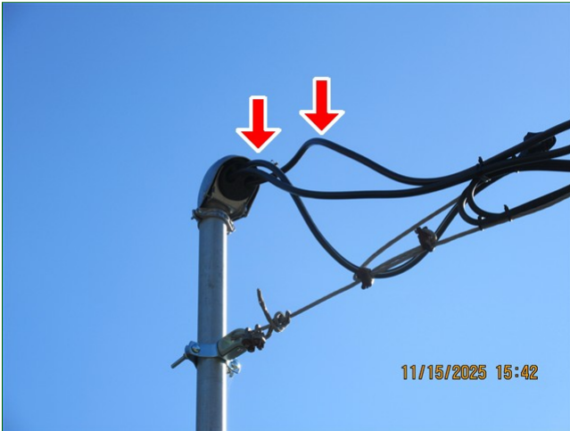
A. Item 3 (Picture) Front left of home, main electric service mast, insufficient drip loop
