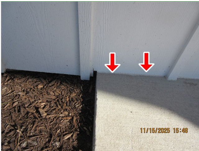
E. Item 14 (Picture) Front of home, cement fiber siding, in direct contact with concrete
