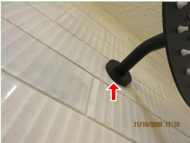
E. Item 28 (Picture) Master bathroom, shower, fixture connections, no sealant
