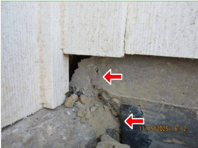
A. Item 3 (Picture) Back of home, foundation, evidence of separate concrete slabs
