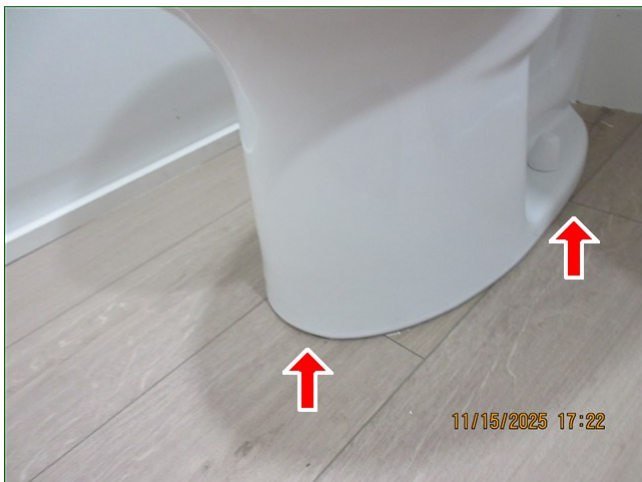
B. Item 3 (Picture) bathroom, toilet floor connection, missing sealant
