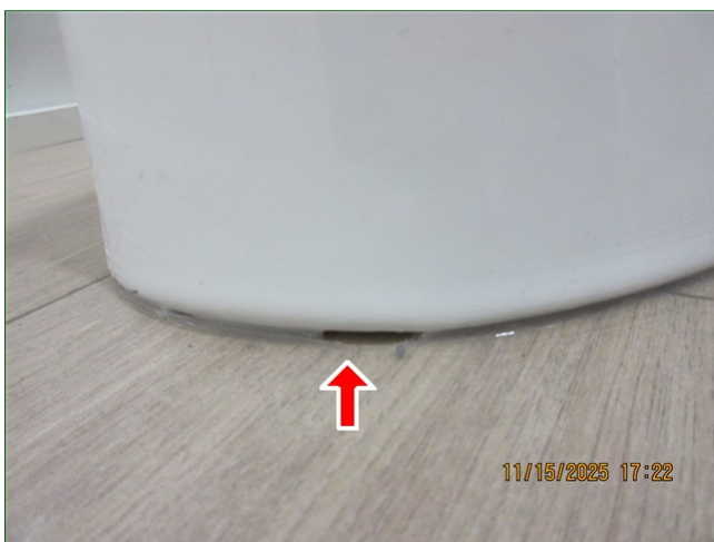
B. Item 4 (Picture) bathroom, toilet floor connection, missing sealant
