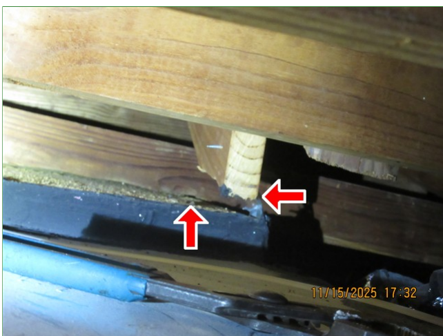
D. Item 8 (Picture) Attic, structural load bearing members, cut
