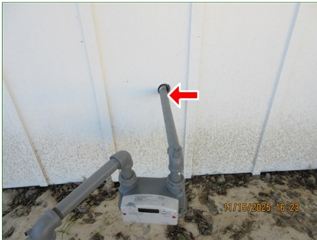
E. Item 2 (Picture) Back of home, gas meter, no electrical bonding wired connection clamp
