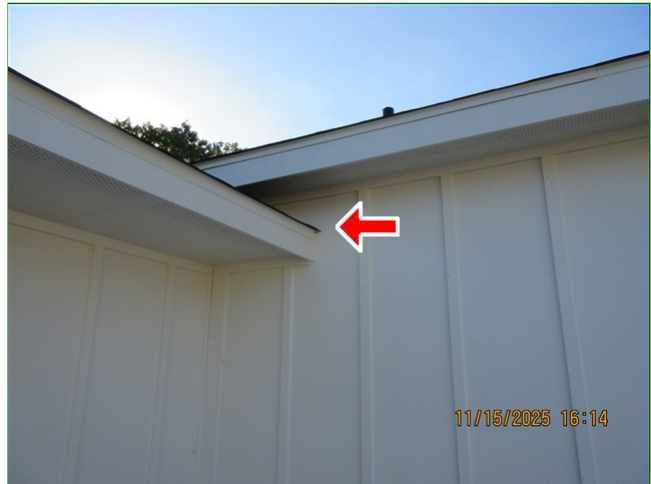
B. Item 6 (Picture) Back of home, roof to wall connection, no kick out flashing
