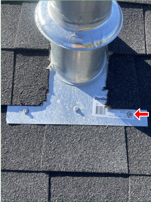
C. Item 1 (Picture) Roof, through roof flashing, exposed nails
