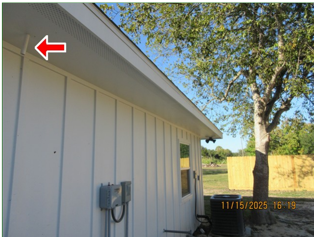
D. Item 1 (Picture) Back of home, condensate drain termination, not in conspicuous location
