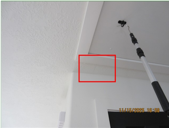
F. Item 1 (Picture) Hallway, ceiling near attic pull down stairs, ceiling, cracked
