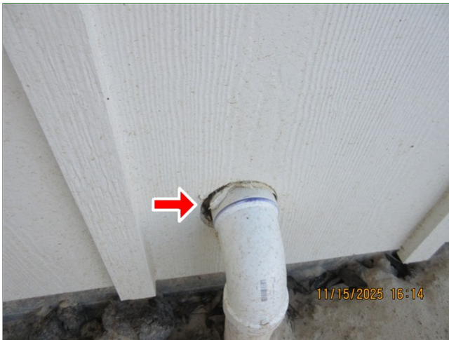
E. Item 20 (Picture) Back of home, through wall termination, no flashing
