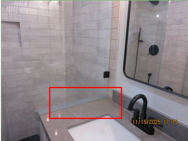
E. Item 29 (Picture) Master bathroom, glass shower wall, missing sealant
