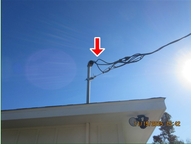
A. Item 2 (Picture) Front left of home, main electric service mast, insufficient drip loop
