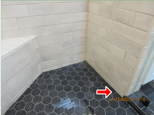
E. Item 26 (Picture) Master bathroom, shower tile wall to floor connection, missing grout
