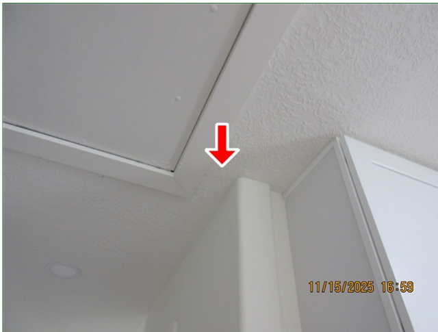
F. Item 4 (Picture) Hallway, ceiling near attic pull down stairs, ceiling, cracked
