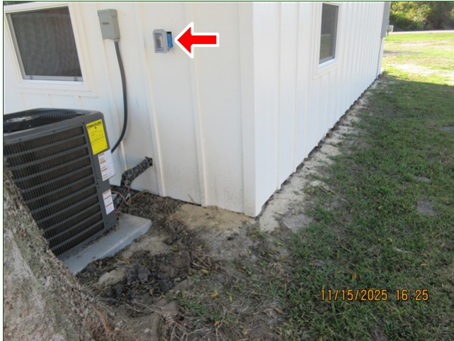
B. Item 1 (Picture) Back of home, electrical outlet box, loose
