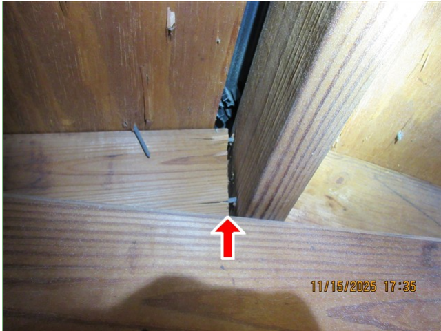
D. Item 4 (Picture) Attic, rafters connection to ridge board, separated
