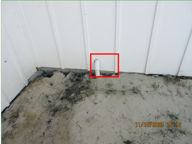
E. Item 19 (Picture) Back of home, through wall termination, no flashing
