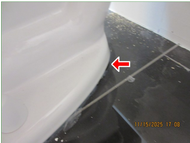
B. Item 2 (Picture) Master bathroom, toilet floor connection, missing sealant
