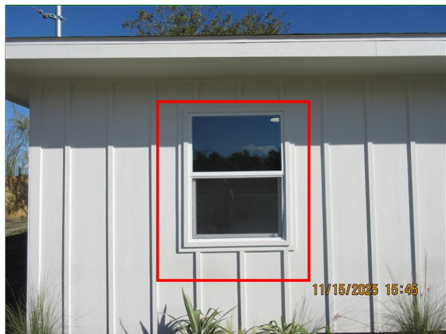
E. Item 11 (Picture) Front of home, cement fiber siding & window butt joints, no flashing
