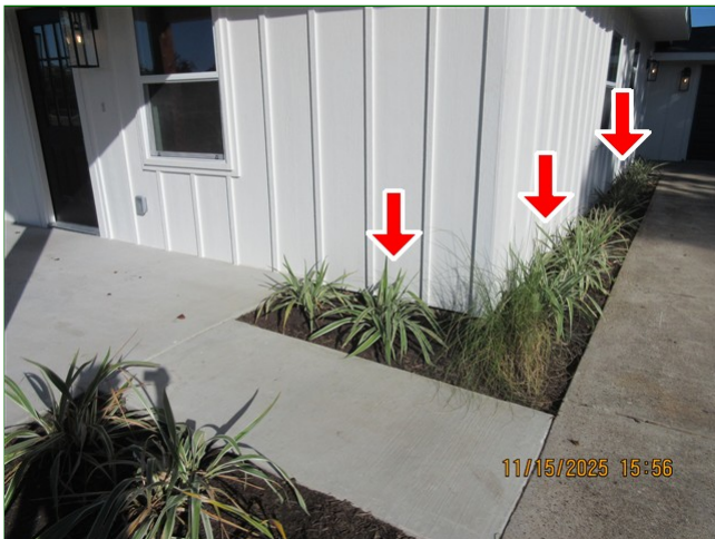
E. Item 1 (Picture) Front and right sides of home, vegetation in direct contact with siding
