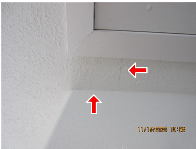
F. Item 2 (Picture) Hallway, ceiling near attic pull down stairs, ceiling, cracked
