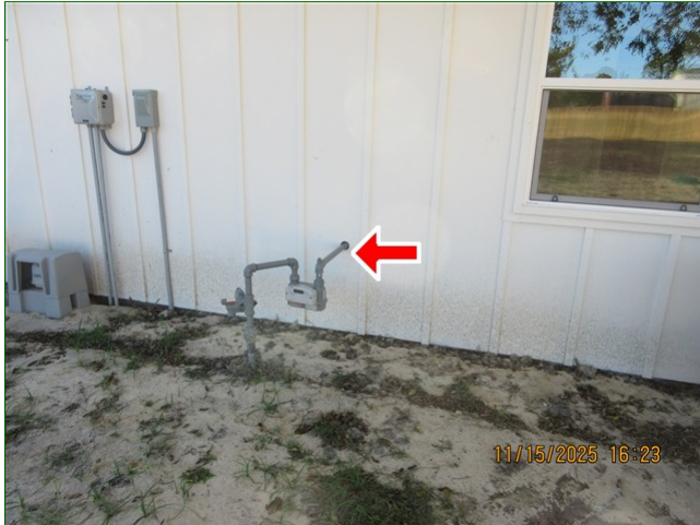
E. Item 1 (Picture) Back of home, gas meter, no electrical bonding wired connection clamp
