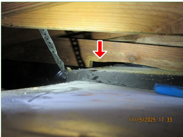
D. Item 7 (Picture) Attic, structural load bearing members, cut
