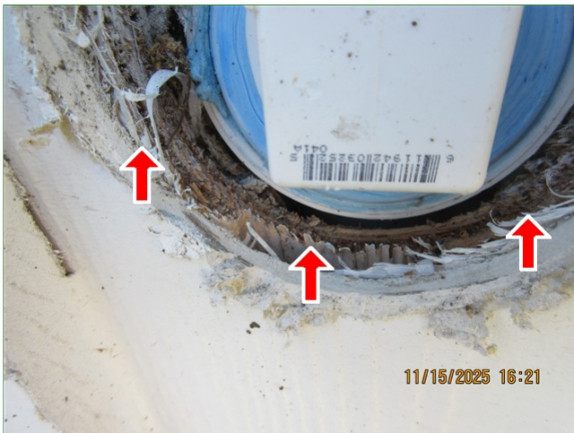
E. Item 25 (Picture) Back of home, through wall termination, no flashing, possible 2 layers of exterior siding
