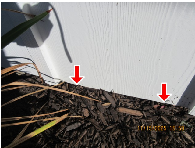
B. Item 5 (Picture) Right of home, high soil/ mulch levels
