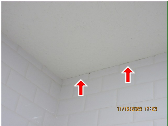
E. Item 10 (Picture) Guest bathroom, tile wall, poor caulk/ sealant work
