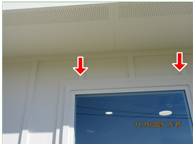
E. Item 12 (Picture) Front of home, cement fiber siding & window butt joints, no flashing
