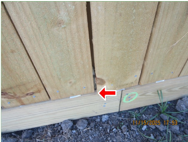
L. Item 2 (Picture) Back of home, fence plank boards, loose
