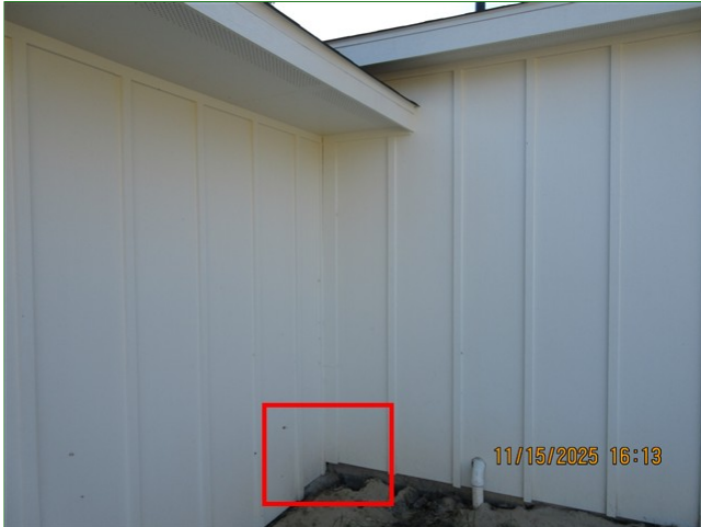
A. Item 1 (Picture) Back of home, foundation, evidence of separate concrete slabs
