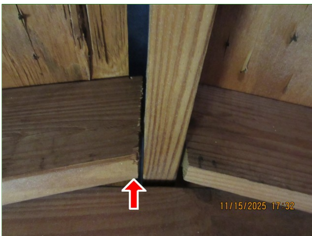
D. Item 3 (Picture) Attic, rafters connection to ridge board, separated
