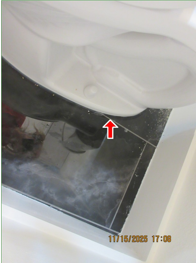
B. Item 1 (Picture) Master bathroom, toilet floor connection, missing sealant
