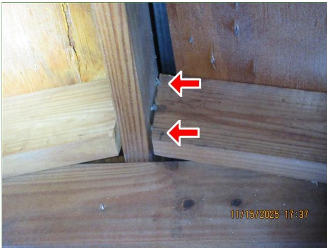
D. Item 5 (Picture) Attic, rafters connection to ridge board, separated
