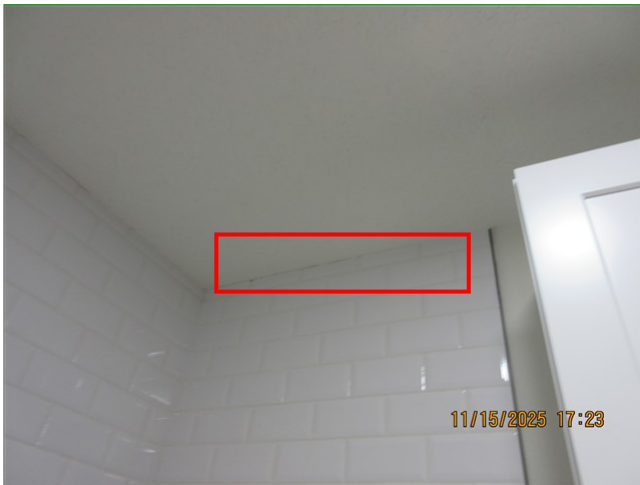
E. Item 8 (Picture) Guest bathroom, tile wall, poor caulk/ sealant work
