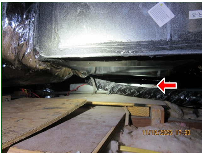
D. Item 2 (Picture) Attic, HVAC unit, insufficient drip pan
