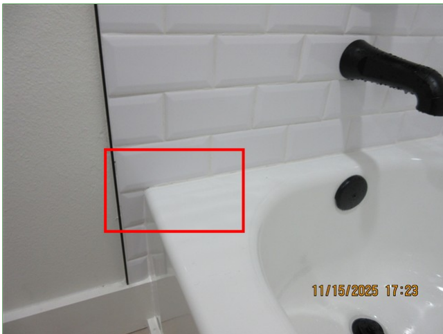
E. Item 31 (Picture) Guest bathroom, tile wall, grout cracked
