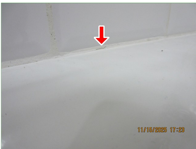
E. Item 33 (Picture) Guest bathroom, tile wall, grout cracked
