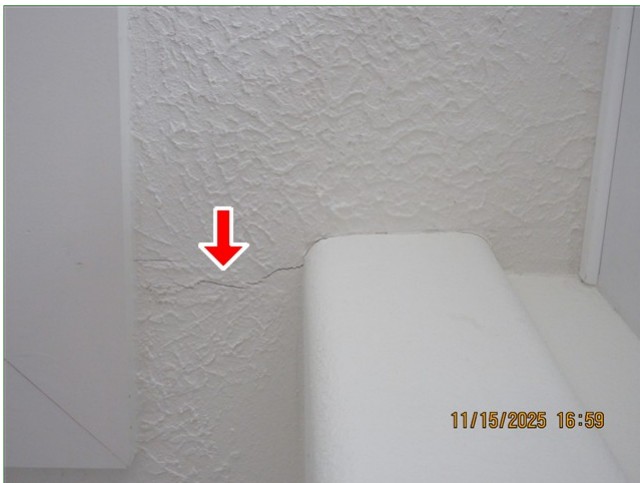
F. Item 5 (Picture) Hallway, ceiling near attic pull down stairs, ceiling, cracked
