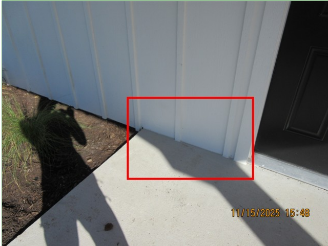
E. Item 13 (Picture) Front of home, cement fiber siding, in direct contact with concrete
