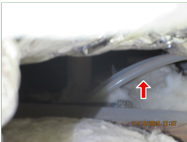
A. Item 1 (Picture) Attic, plumbing supply pipes, exposed
