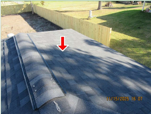
D. Item 1 (Picture) Garage, roof decking, soft spots
