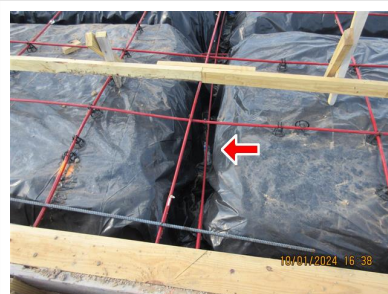
2.3 Item 13 (Picture) Exterior footing "wall", trash
