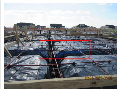
2.3 Item 3 (Picture) Vapor barrier, tears and gaps/ separation
