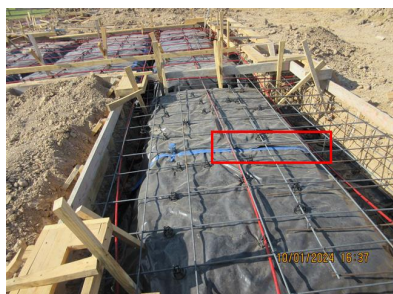
2.3 Item 7 (Picture) Vapor barrier, tears and gaps/ separation
