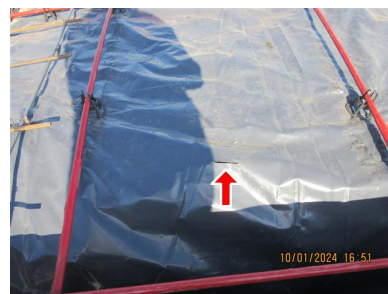
2.3 Item 9 (Picture) Vapor barrier, tears and gaps/ separation
