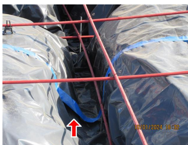
2.3 Item 2 (Picture) Vapor barrier, tears and gaps/ separation
