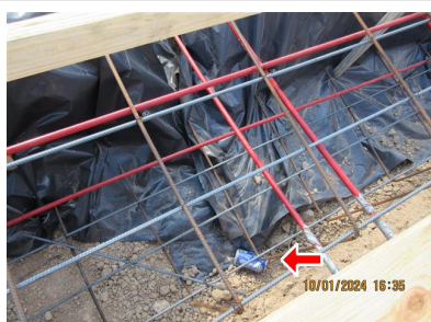
2.3 Item 11 (Picture) Exterior footing "wall", trash
