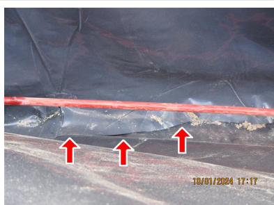
2.3 Item 10 (Picture) Vapor barrier, tears and gaps/ separation
