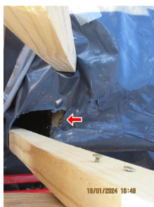
2.3 Item 8 (Picture) Vapor barrier, tears and gaps/ separation
