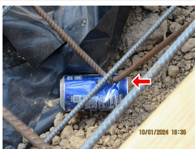
2.3 Item 12 (Picture) Exterior footing "wall", trash
