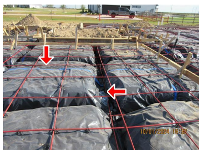
2.3 Item 1 (Picture) Vapor barrier, tears and gaps/ separation
