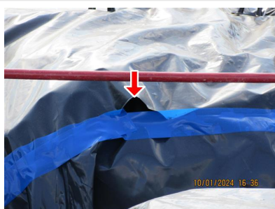
2.3 Item 4 (Picture) Vapor barrier, tears and gaps/ separation
