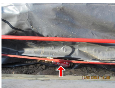
2.3 Item 15 (Picture) Exterior footing "wall", trash
