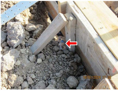
2.3 Item 17 (Picture) Exterior footing "wall", trash
