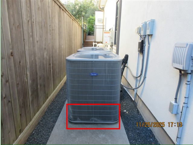
B. Item 3 (Picture) Left of home, condenser coils, damaged
