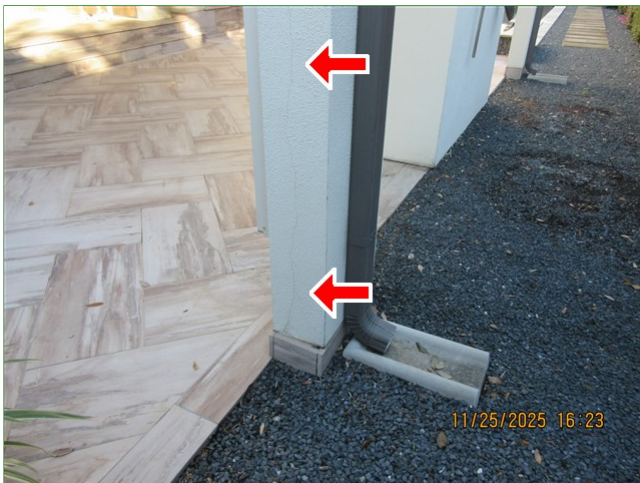
E. Item 9 (Picture) Back of home, stucco siding, hairline cracks
