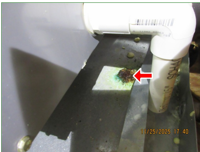
D. Item 2 (Picture) Attic, HVAC refrigerant line, small drip leak
