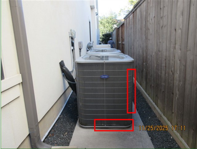
B. Item 1 (Picture) Left of home, condenser coils, damaged
