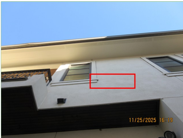
E. Item 3 (Picture) Right of home, stucco siding, hairline crack
