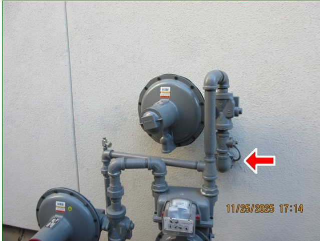
E. Item 1 (Picture) Left of home, gas meter, supply line bonding clamp, rusted and painted
