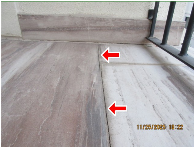
K. Item 2 (Picture) Second story, balcony, tile floor covering, grout/ mortar, normal wear & tear
