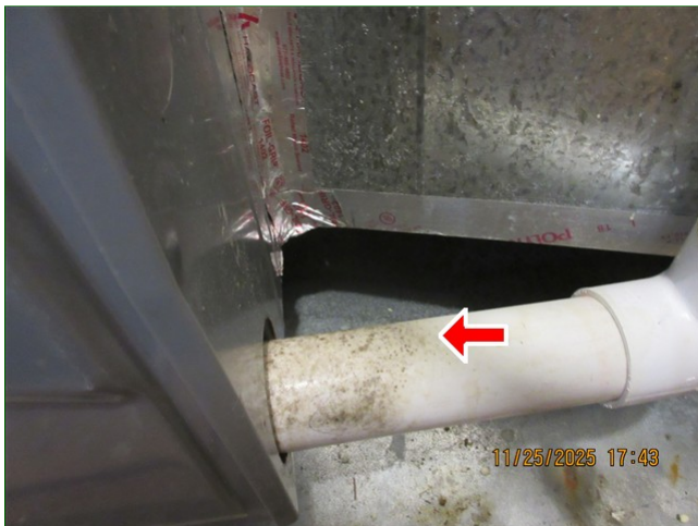
C. Item 3 (Picture) Attic, furnace vent pipe, potential organic growth
