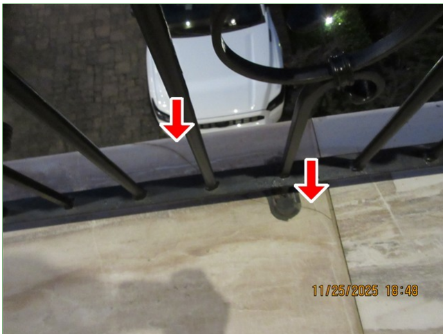
K. Item 3 (Picture) Second story, balcony above garage, tile floor covering, cracked
