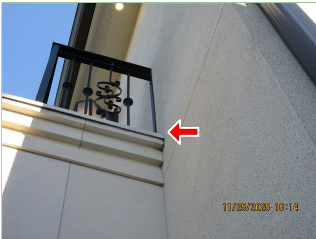
E. Item 6 (Picture) Front of home, balcony to wall connection, no kick-out flashing
