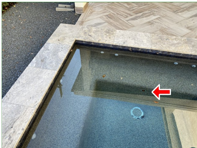
T. Item 1 (Picture) Hot tub, light, not functioning & possible rust build up
