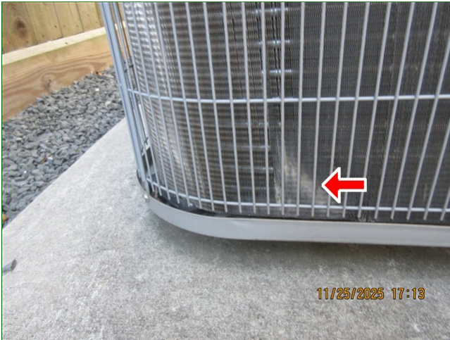
B. Item 4 (Picture) Left of home, condenser coils, damaged
