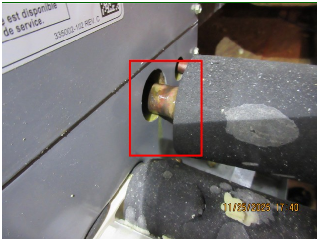
D. Item 1 (Picture) Attic, HVAC refrigerant line, small drip leak
