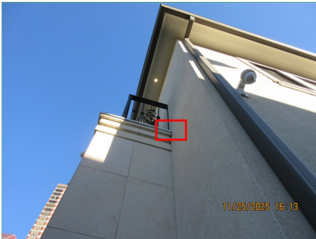
E. Item 5 (Picture) Front of home, balcony to wall connection, no kick-out flashing
