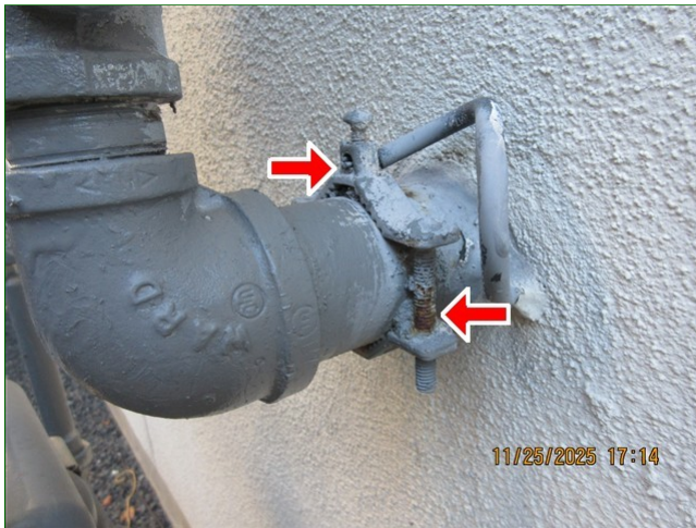
E. Item 2 (Picture) Left of home, gas meter, supply line bonding clamp, rusted and painted
