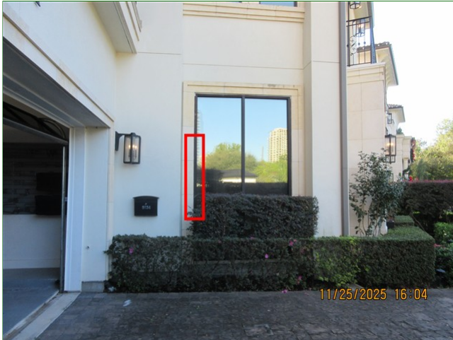
H. Item 1 (Picture) Front of home, window to stone trim butt joint connections, caulk/ sealant, normal wear & tear
