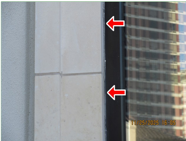
H. Item 2 (Picture) Front of home, window to stone trim butt joint connections, caulk/ sealant, normal wear & tear
