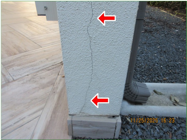
E. Item 10 (Picture) Back of home, stucco siding, hairline cracks
