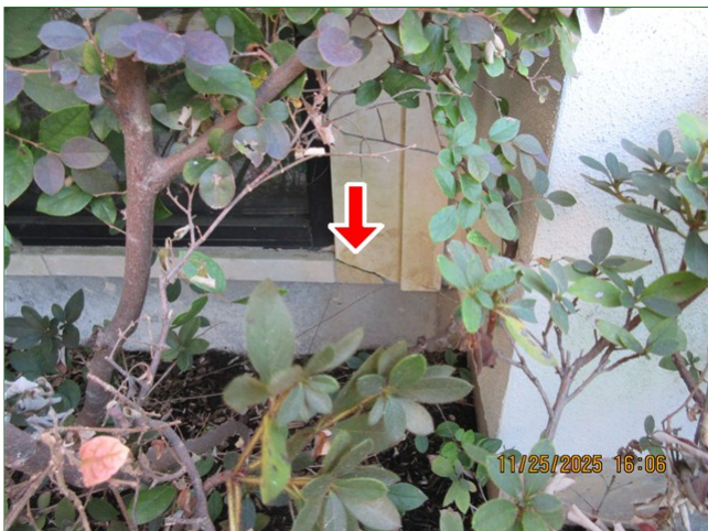
H. Item 3 (Picture) Front of home, stone window trim, cracked
