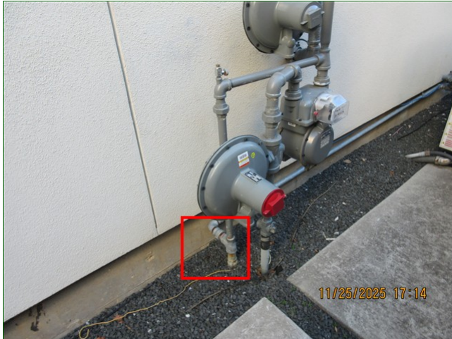
E. Item 3 (Picture) Left of home, gas meter, supply line connections, rust
