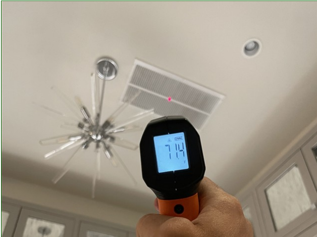
B. Item 5 (Picture) Common area, HVAC return vent, temp. reading
