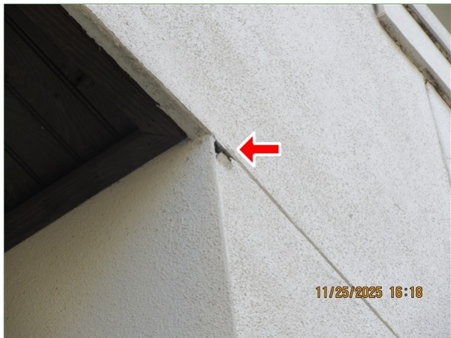
E. Item 14 (Picture) Right of home, stucco siding, damaged
