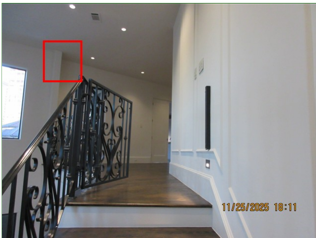
F. Item 1 (Picture) Second story, ceiling, minor hairline cracks
