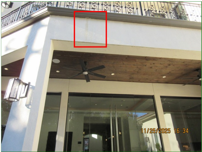
E. Item 11 (Picture) Back of home, stucco siding, moisture stains
