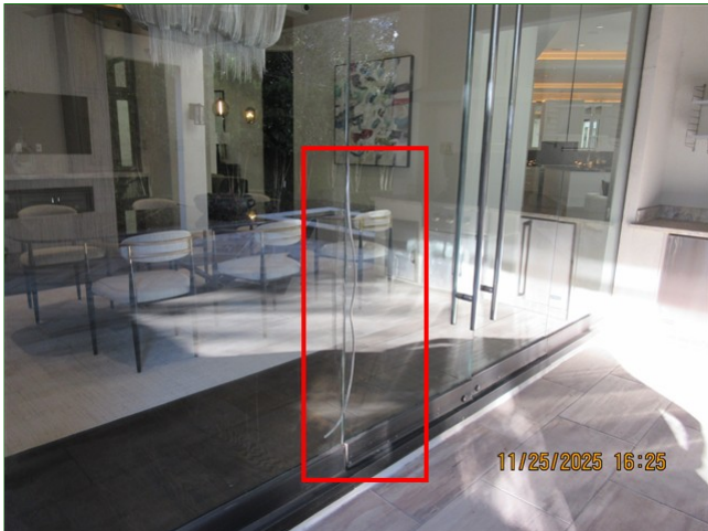
G. Item 1 (Picture) Back of home, exterior door, loose weather stripping
