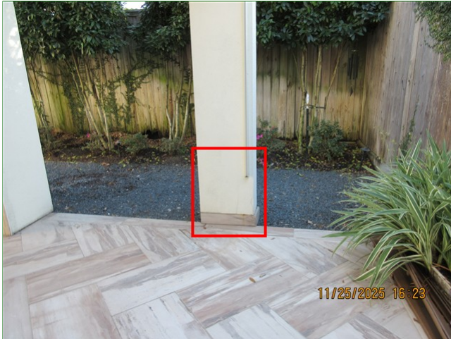
E. Item 1 (Picture) Back of home, stucco siding, hairline cracks
