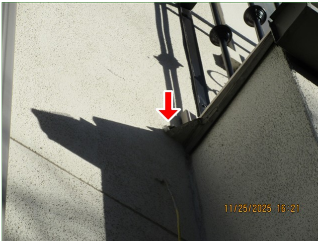
E. Item 8 (Picture) Right of home, balcony to wall connection, non standard kick-out flashing
