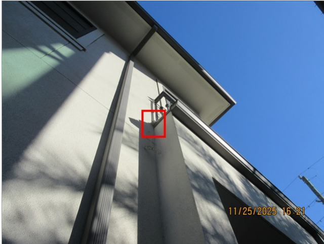
E. Item 7 (Picture) Right of home, balcony to wall connection, non standard kick-out flashing
